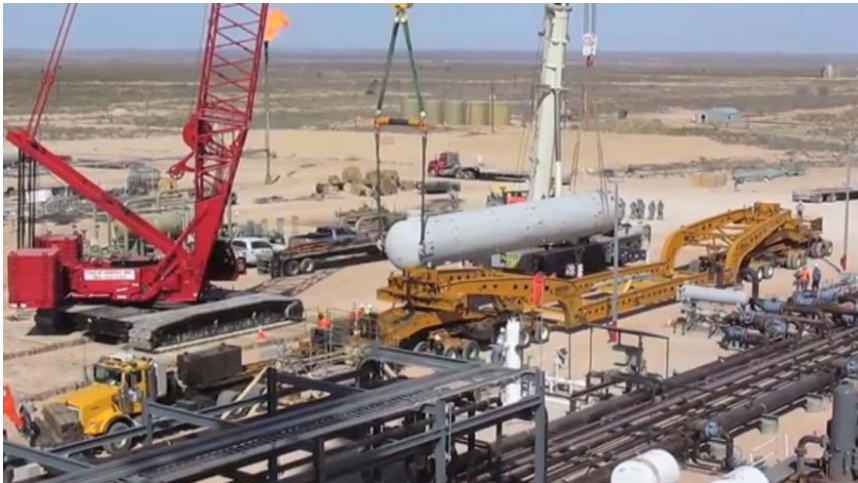
Saulsbury Industries Vessel Lift
