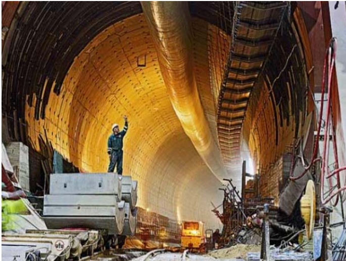
Yangtze River Tunnels, China
