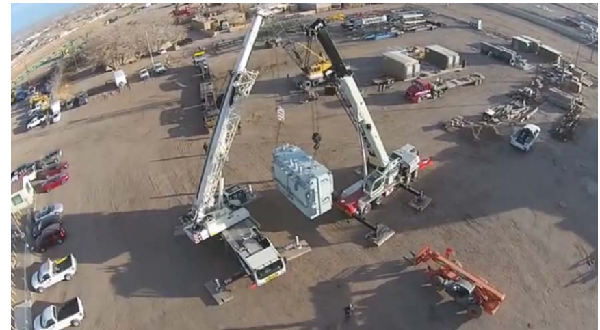
122,000lb Transformer Lift
