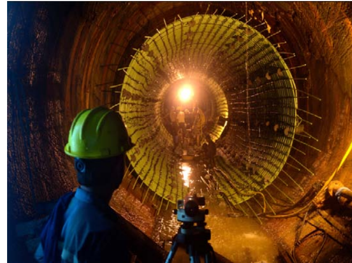
HCC's Maroshi-Ruparel water tunnel project in Mumbai
